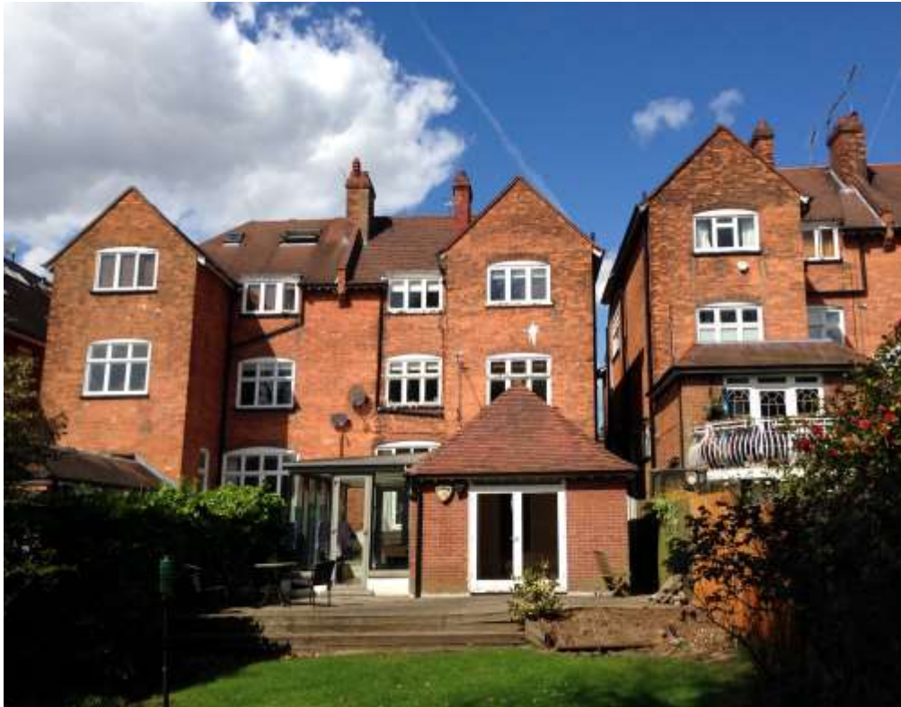
Fig 1: View of rear elevation
