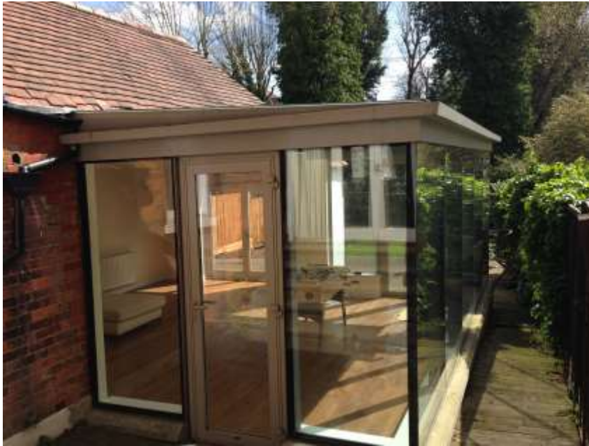
Fig 4: View of existing conservatory
