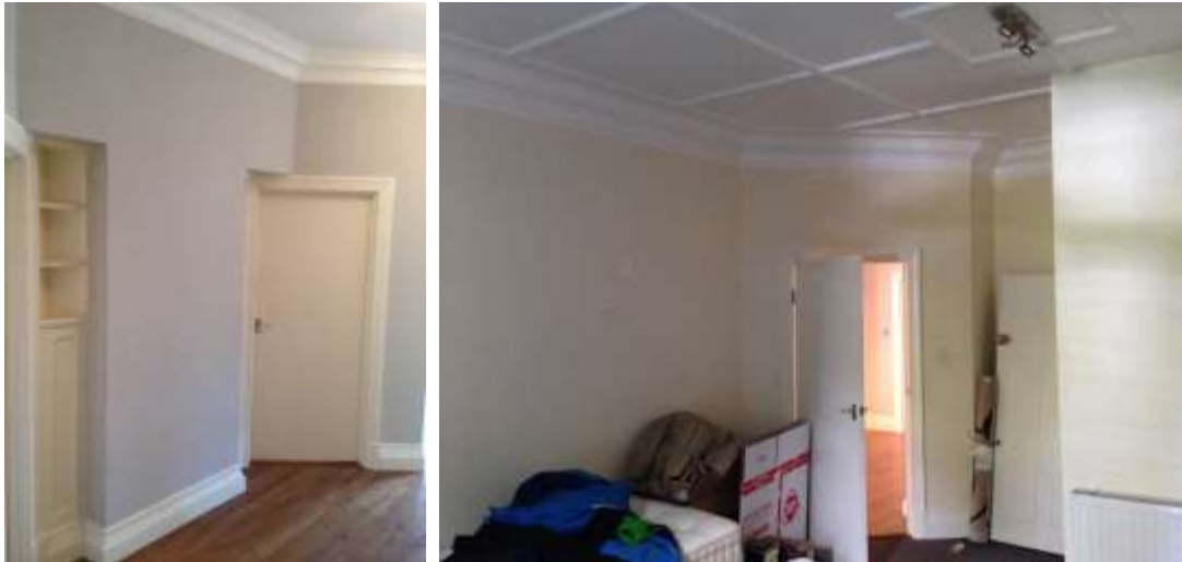
5: Interiors at ground floor
