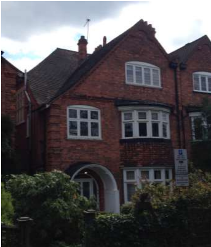
Fig 1: View of front elevation
