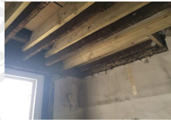
Master Bedroom. Photo showing new floor joists bolted to original
