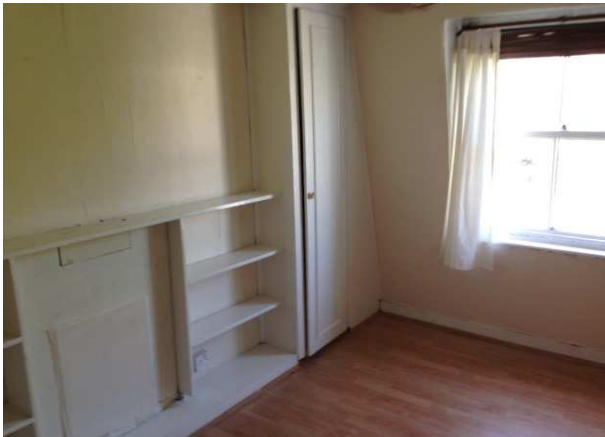
Photo 26 Third floor - Rear Fireplace number :TF 01 Comments: Blocked in
