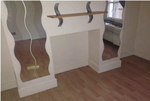
Photo 17 Ground floor - Rear (G 01) Fireplace number: GF 01 Comments: No surround
