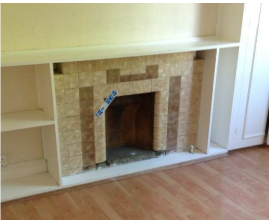
Photo 24 Second floor - Rear (S 01) Fireplace number: SF 02 Comments:
