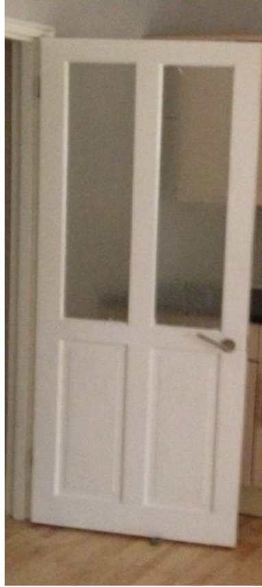
Photo 41 Location: First Floor FD - 01 Comments: Discard
