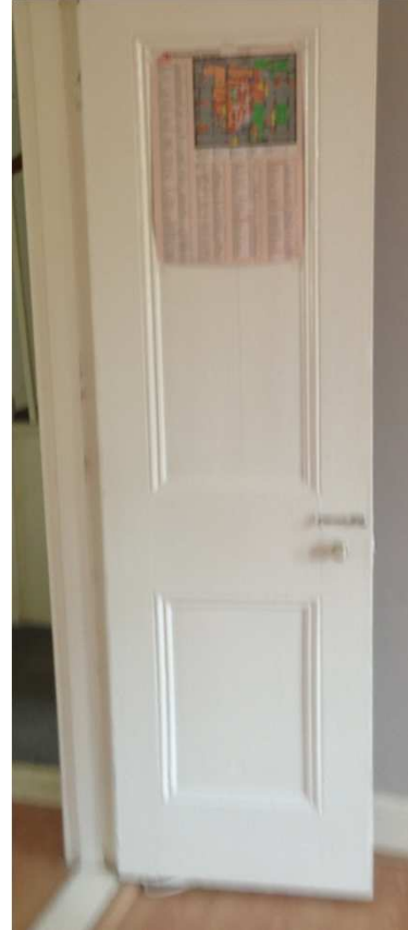
Photo 42 Location: First floor FD - 02 Comments: Reuse in LGD 07
