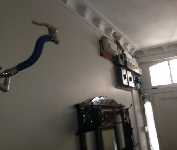
Photo 28 Comments: Re store original cornice.
