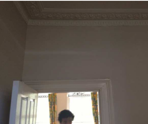
Photo 34 First floor - Rear F -01
