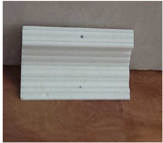
Photo 35 First floor - Rear F -01
