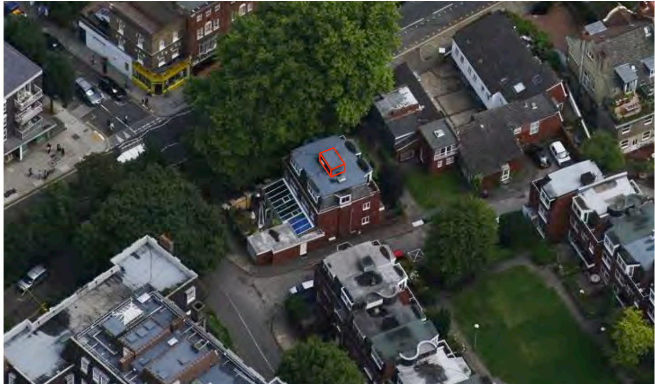
AERIAL VIEW FROM THE WEST
