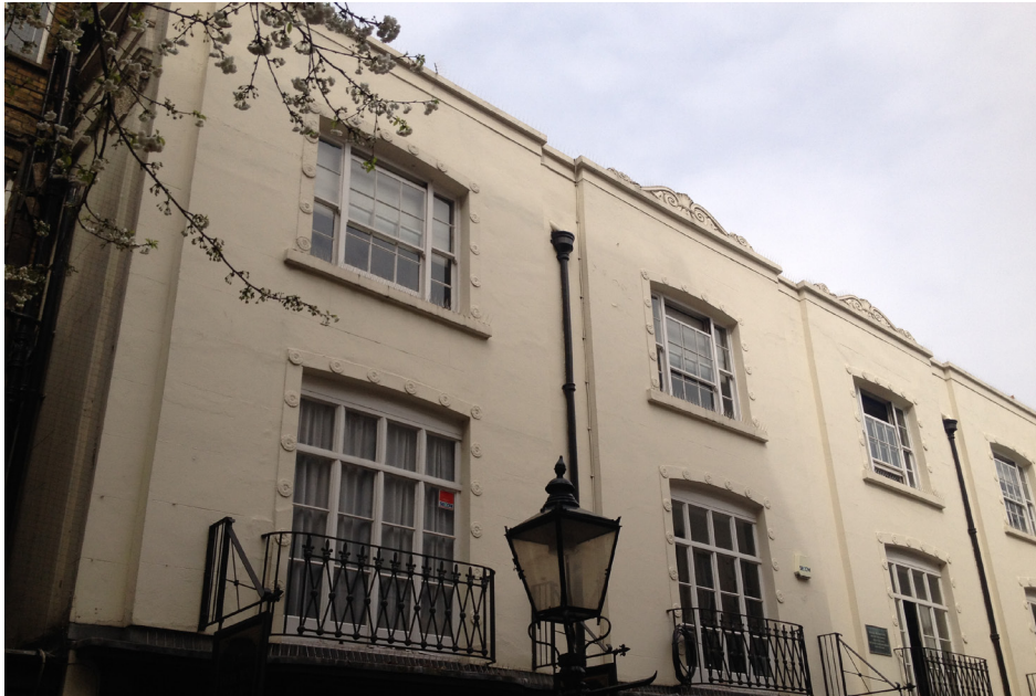
Front façade onto Woburn Walk.
