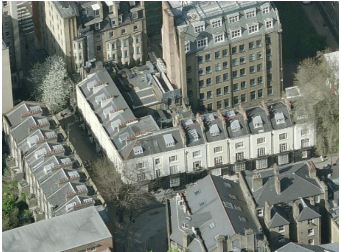
Aerial view looking West over the site.
