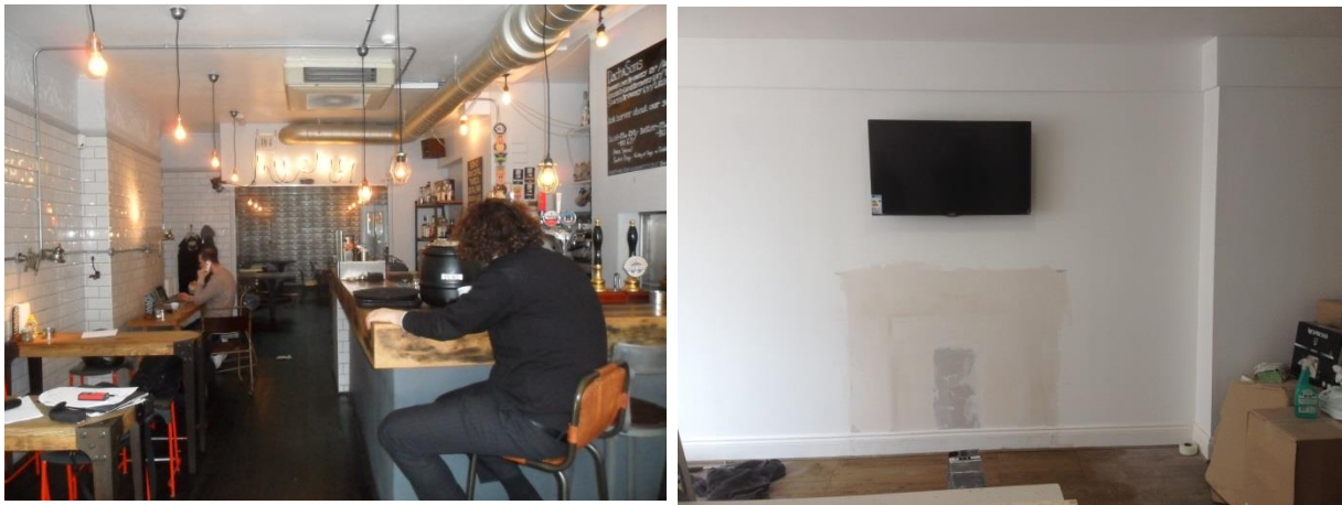
Cornice exposed (previous restaurant) and cornice covered (current estate agency)
