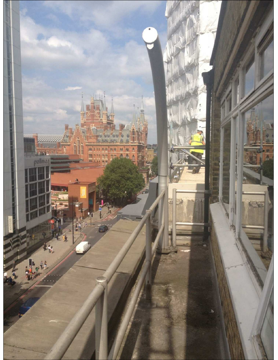
2 076 View of the existing 6th floor roof towards East NTS@A3
