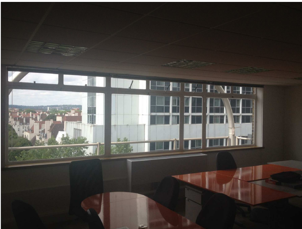
3 076 View of the existing 6th floor roof from the 6th floor office NTS@A3
