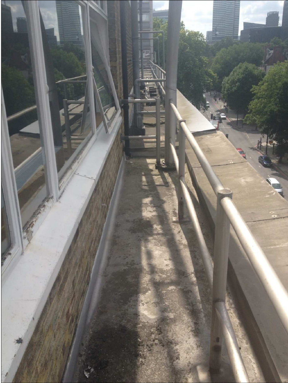
1 076 View of the existing 6th floor roof towards West NTS@A3
