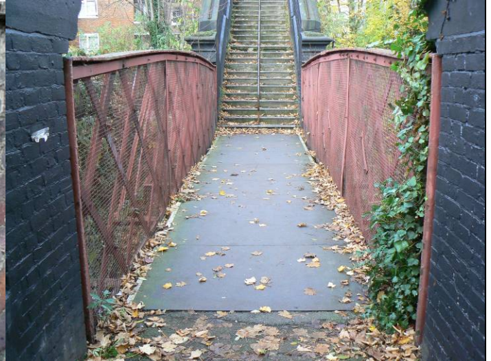
View across footbridge looking north
