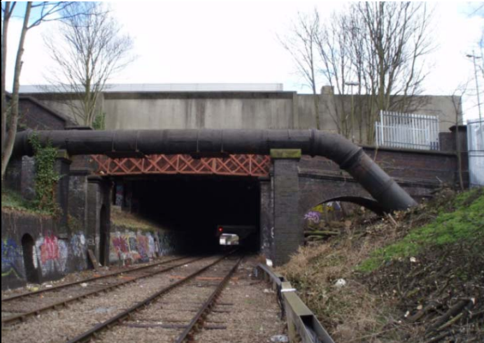
Trackside view looking east
