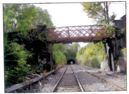
PHOTO OF EAST ELEVATION
