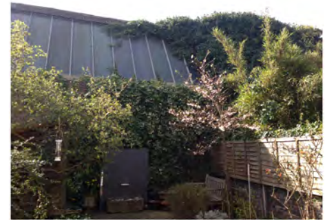
View of existing building from rear of Evangelist Road
