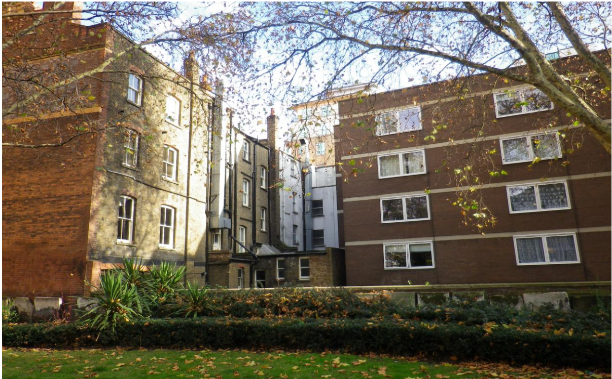
View of Rear of nos. 61-65 St Giles High Street
