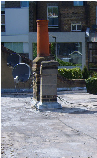
Photo 06 Taller chimney to roof at no 6.
