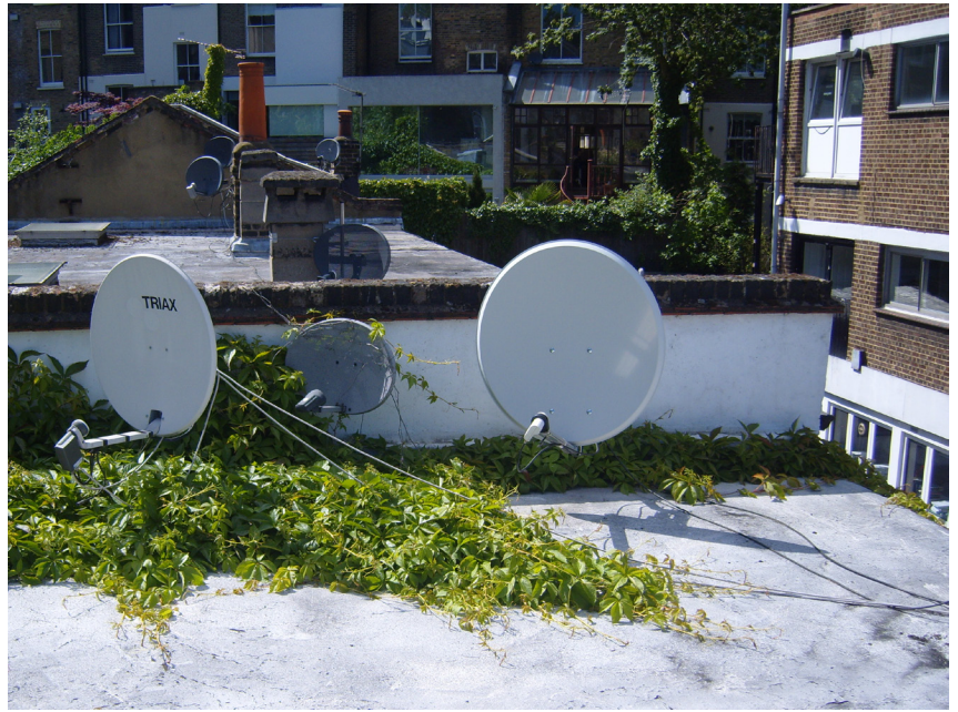
Photo 07 View from roof of no 3 towards nos 5 and 6.
