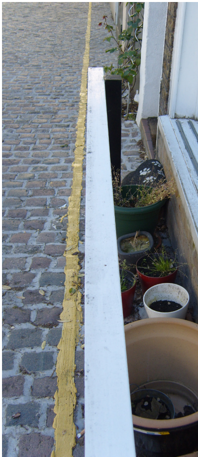
Photo 08 View showing crash barrier and single yellow line in front of no 3.
