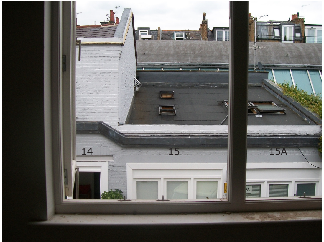
Photo 04 View towards nos 14 (taller building to the very left), 15 and 15A from the 1st fl window opening at no 3 proposed extended downwards.
