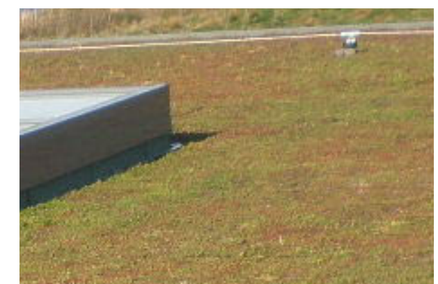
Example of a sedum extensive green roof by Bauder
