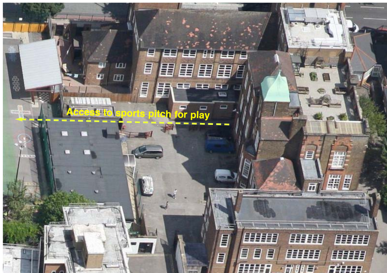
Existing car park in the north courtyard
