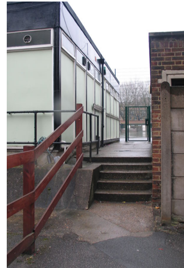
Access to sports pitch, with car park fence
