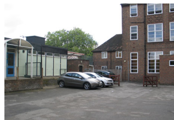
Existing car park, 22.05.14
