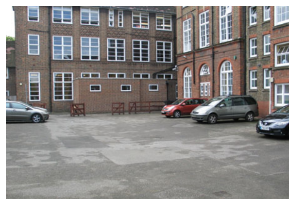
Existing car park, 22.05.14
