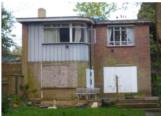
Plate 3.1: Rear of Building 1
