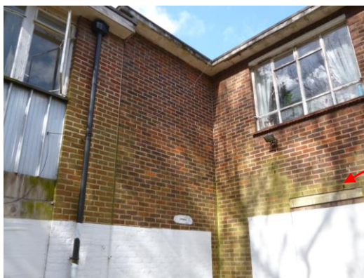
Plate 3.2: Example of weep holes (denoted by red arrow)
