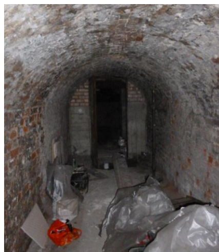
Plate 3.5: Internal view of the tunnel
