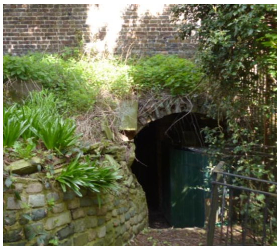
Plate 3.4: External view of tunnel
