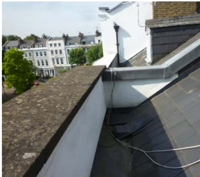
Existing concrete coping parapet to 31 Chalcot Square (32 Chalcot Square beyond)
