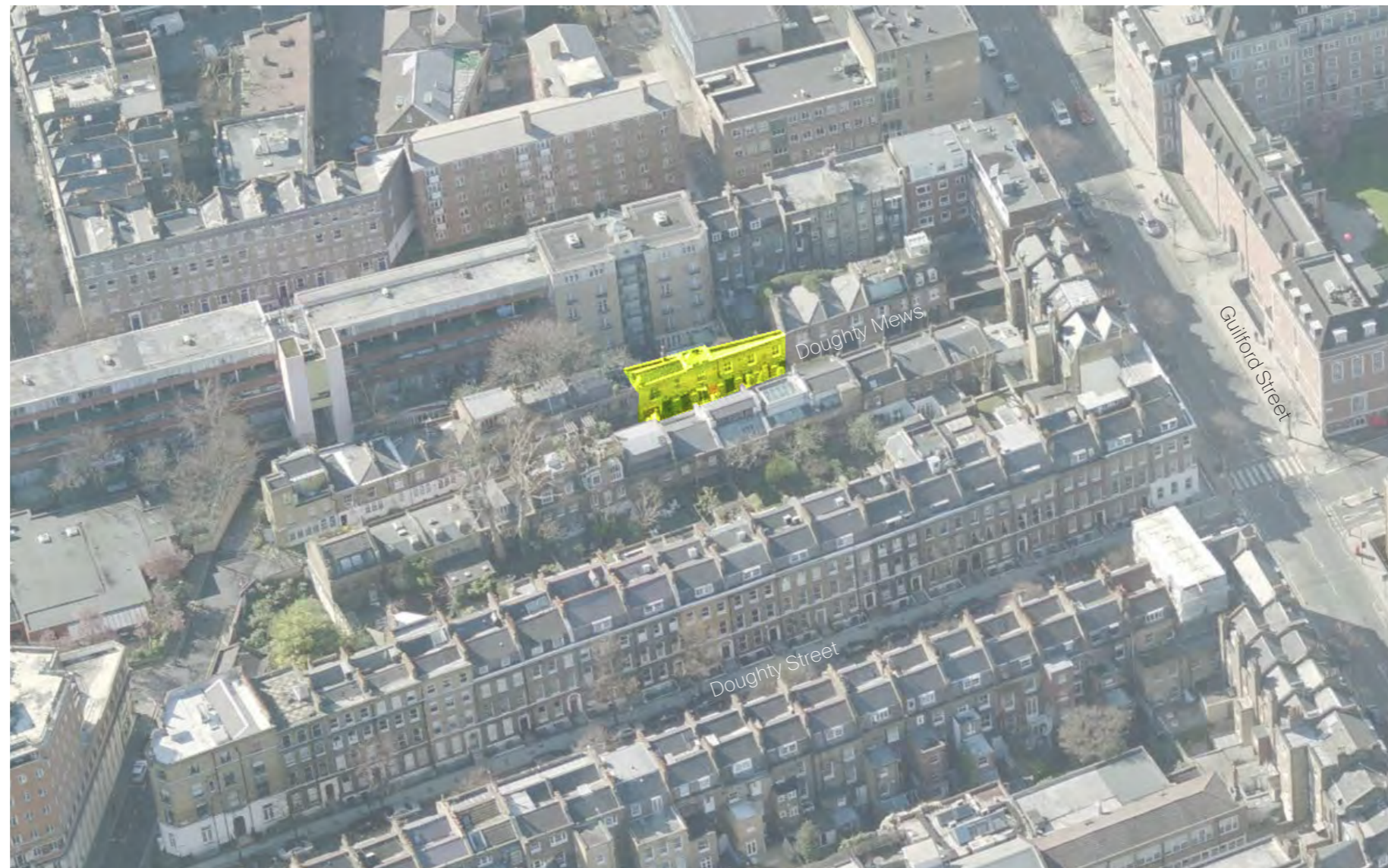
Aerial site photograph highlighting 19 & 20 Doughty Mews
