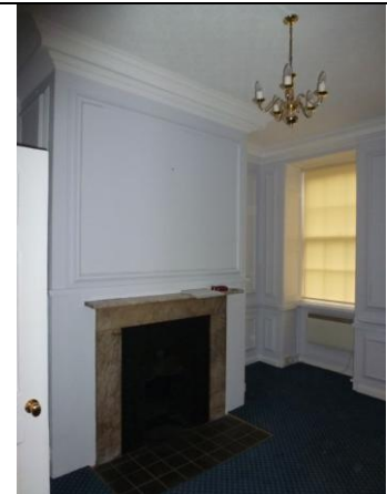
Fig 3 Fireplace and Wall panelling North Office
