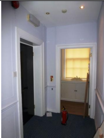
Fig 4 Ground floor Entrance Lobby, Door from Stair and Toilet beyond
