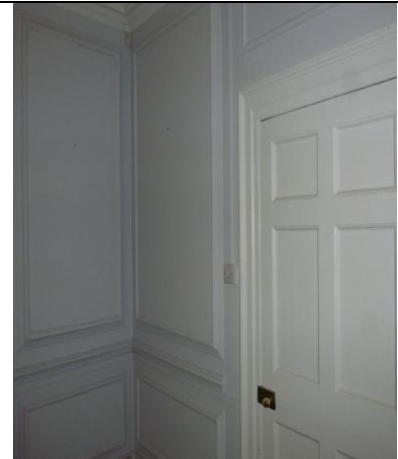
Fig 6 Existing door and wall panelling – North Office
