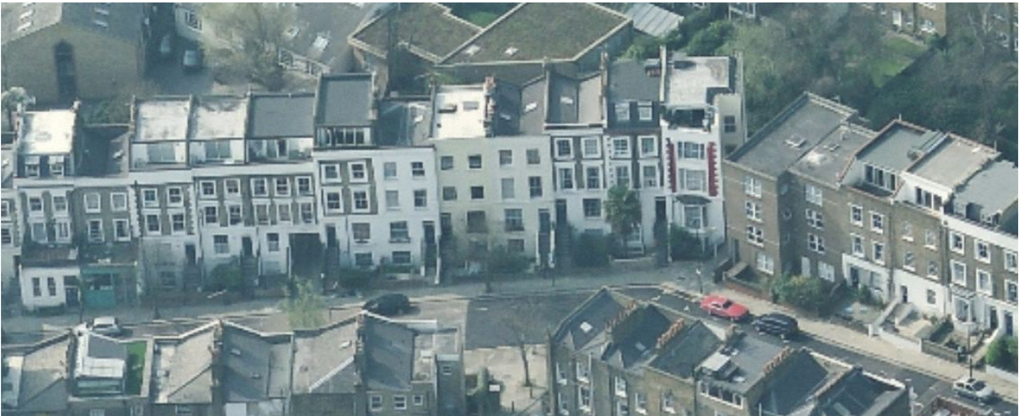
View from East
