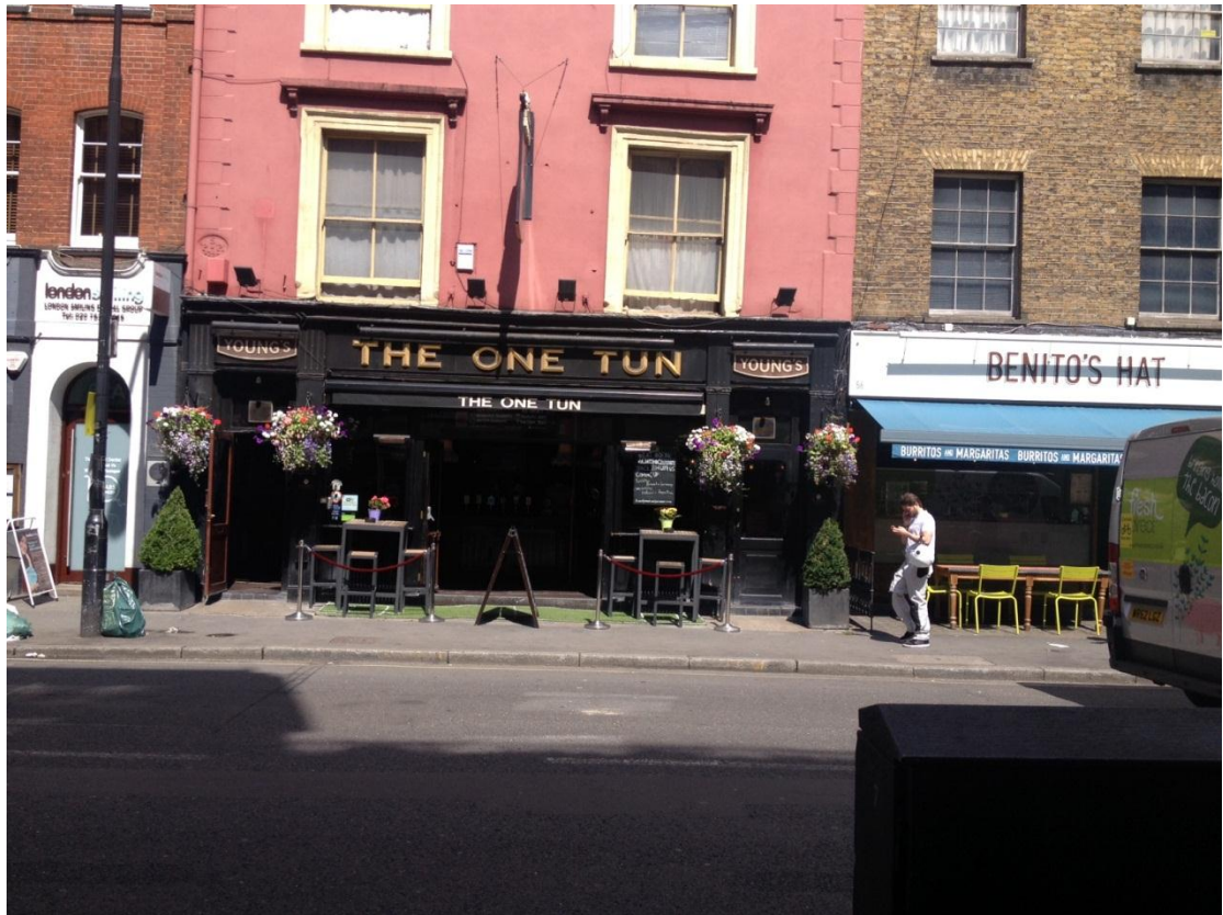
Photo 1- Existing shopfront (with doors open)
