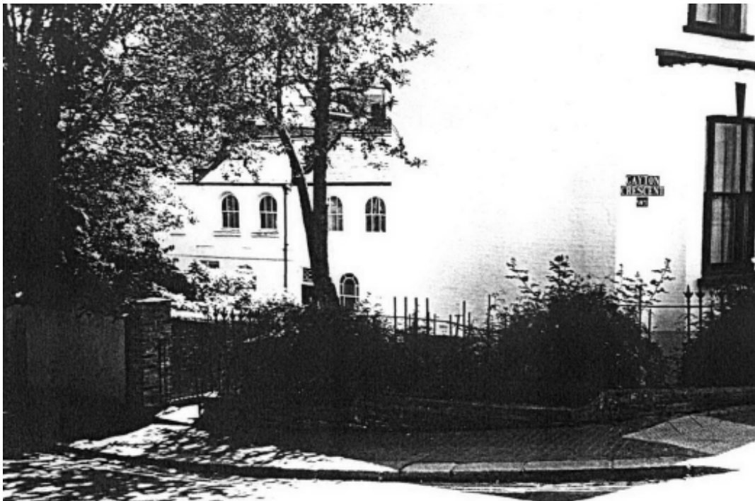
Photo showing railings in situ (taken from previous planning application on property in June 2006)
