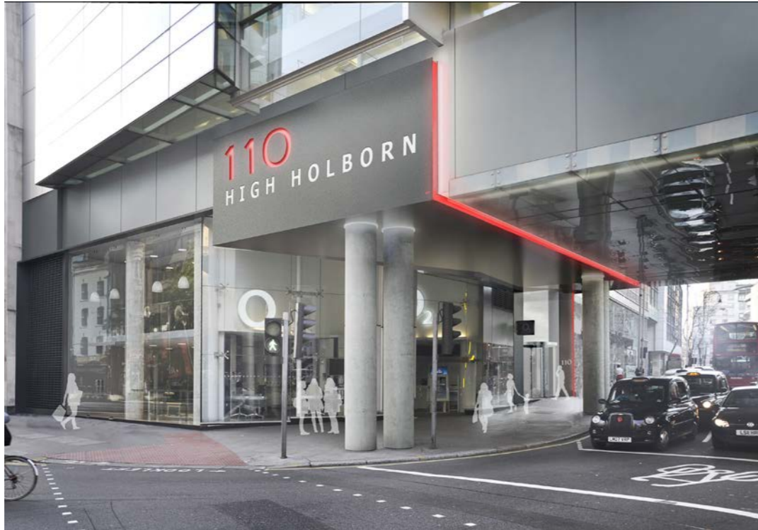
Entrance as approved, with existing single glazed undercroft cladding
