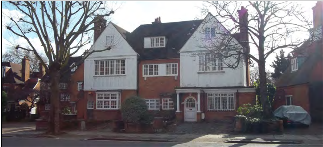
Fig. 2 – Front elevation with the existing porches and dormer and 53 to the left and 53a to the right.
