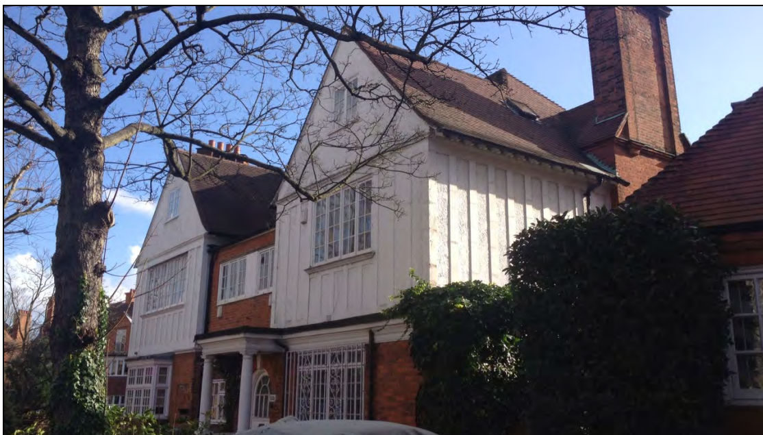
Fig. 4 – Front elevation looking South East with 53a in the foreground
