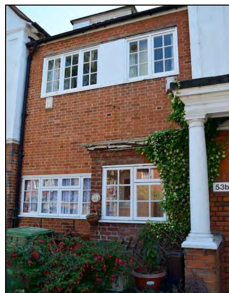
Fig. 9 – Existing 20 th Century porch and altered façade of 53a.
