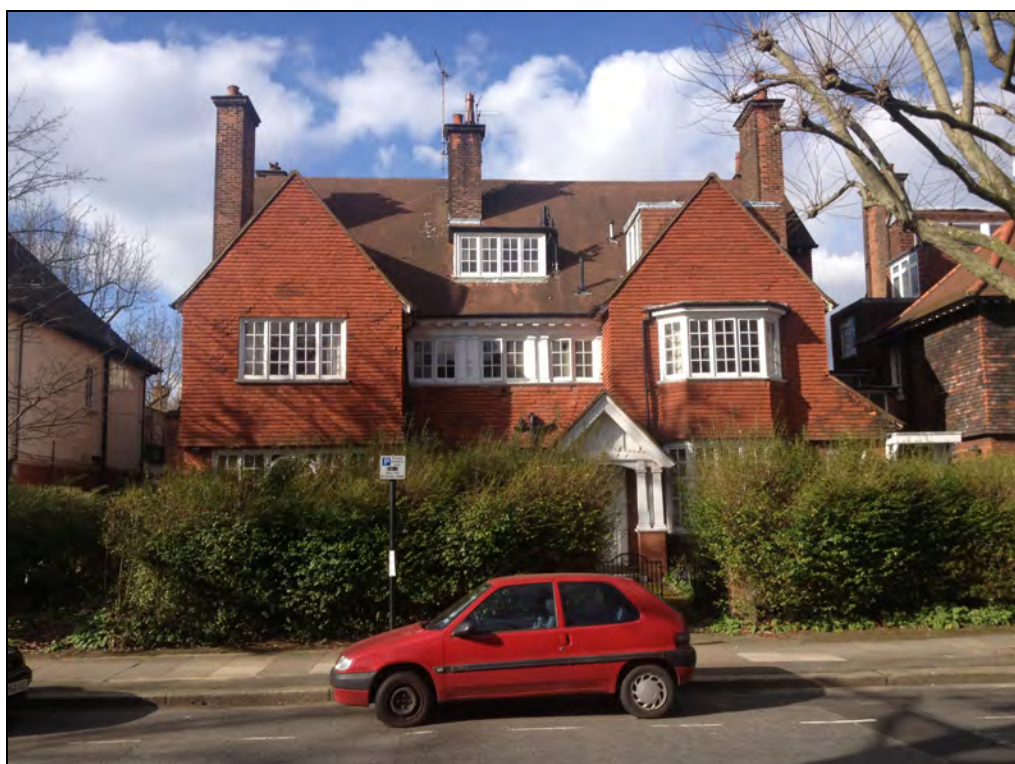
Fig. 12 – No. 56 Elsworthy Road, precedent of similar front elevation for No's 53 and 53a, including central dormer, two storey right-hand bay and porch located between the shallow projecting wings.
