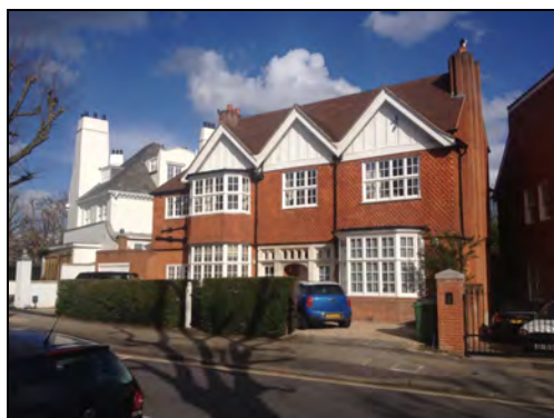
Fig. 10 – No. 2 Wadham Gardens, precedent for double height bays and central doorway
