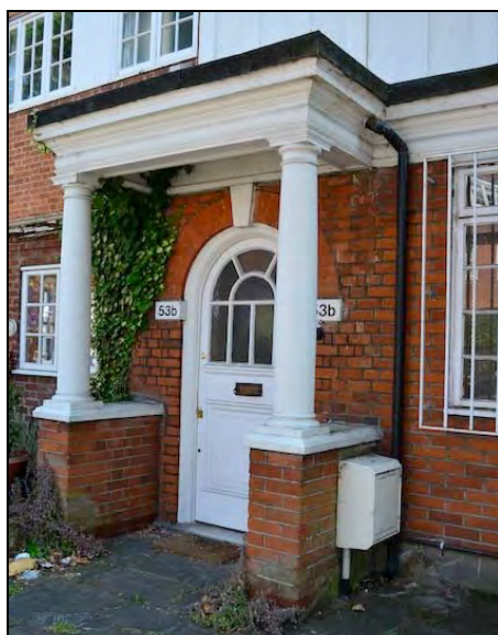
Fig. 8 – Existing porch and entrance door formerly of 53b.
