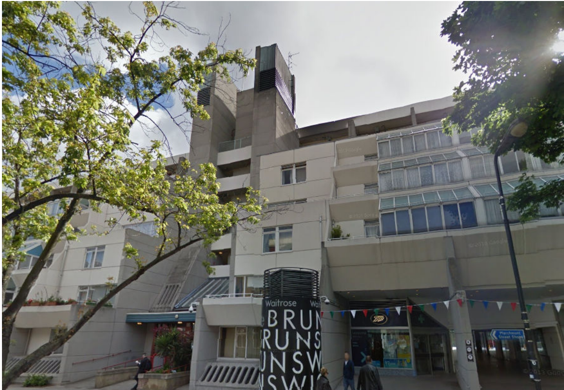
ABOVE: The towers projecting above the Brunswick.
