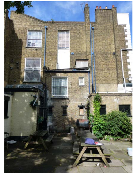
Rear elevation of 101 Brecknock Road
