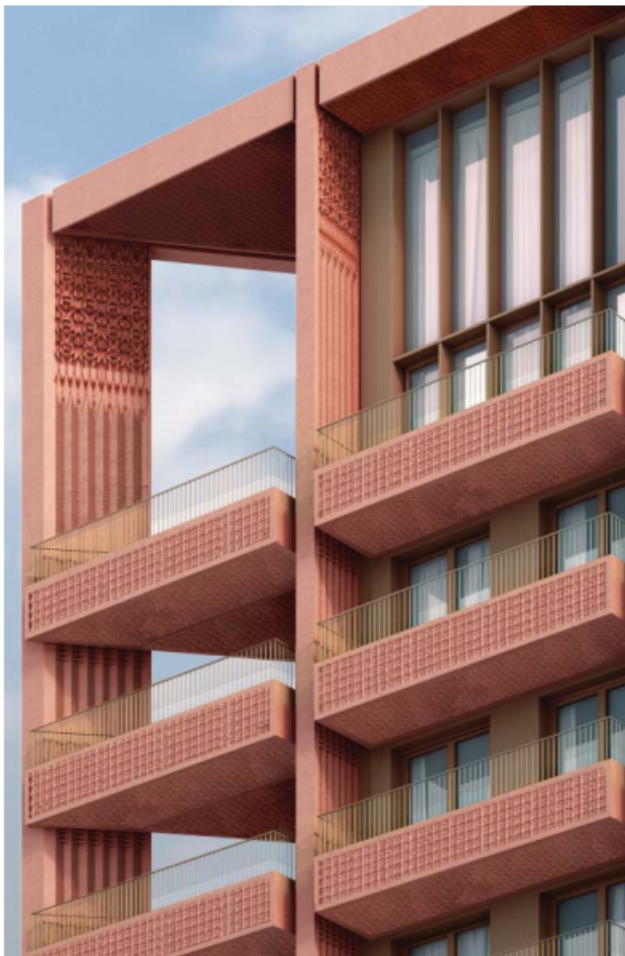
Eastern façade detail
