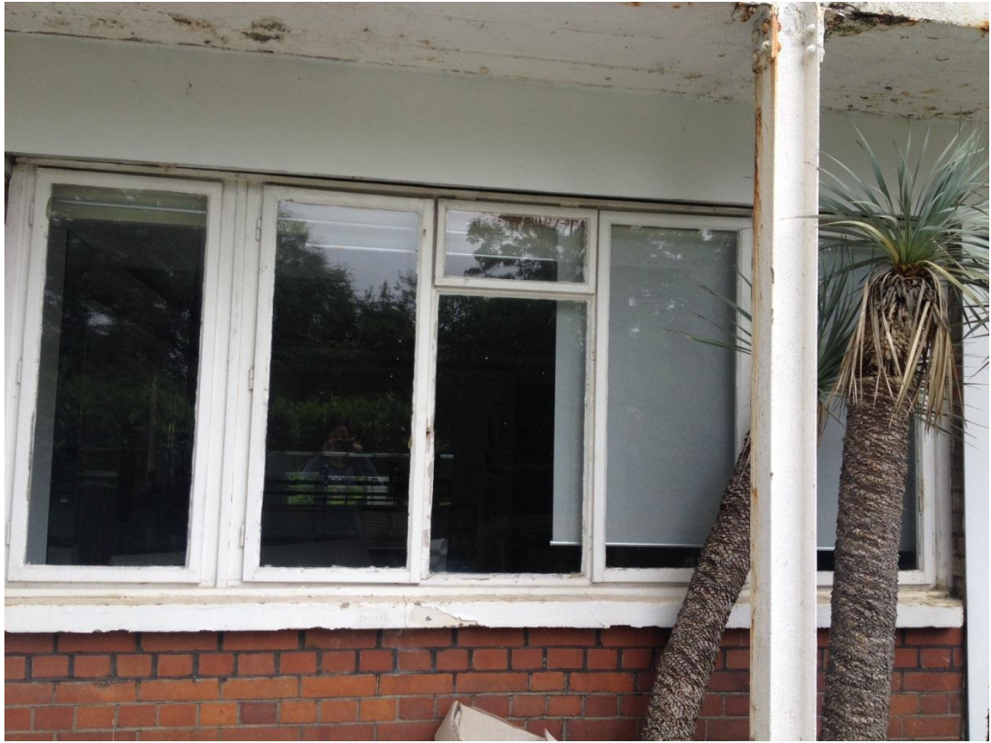
EXISTING REAR ELEVATION WINDOWS
