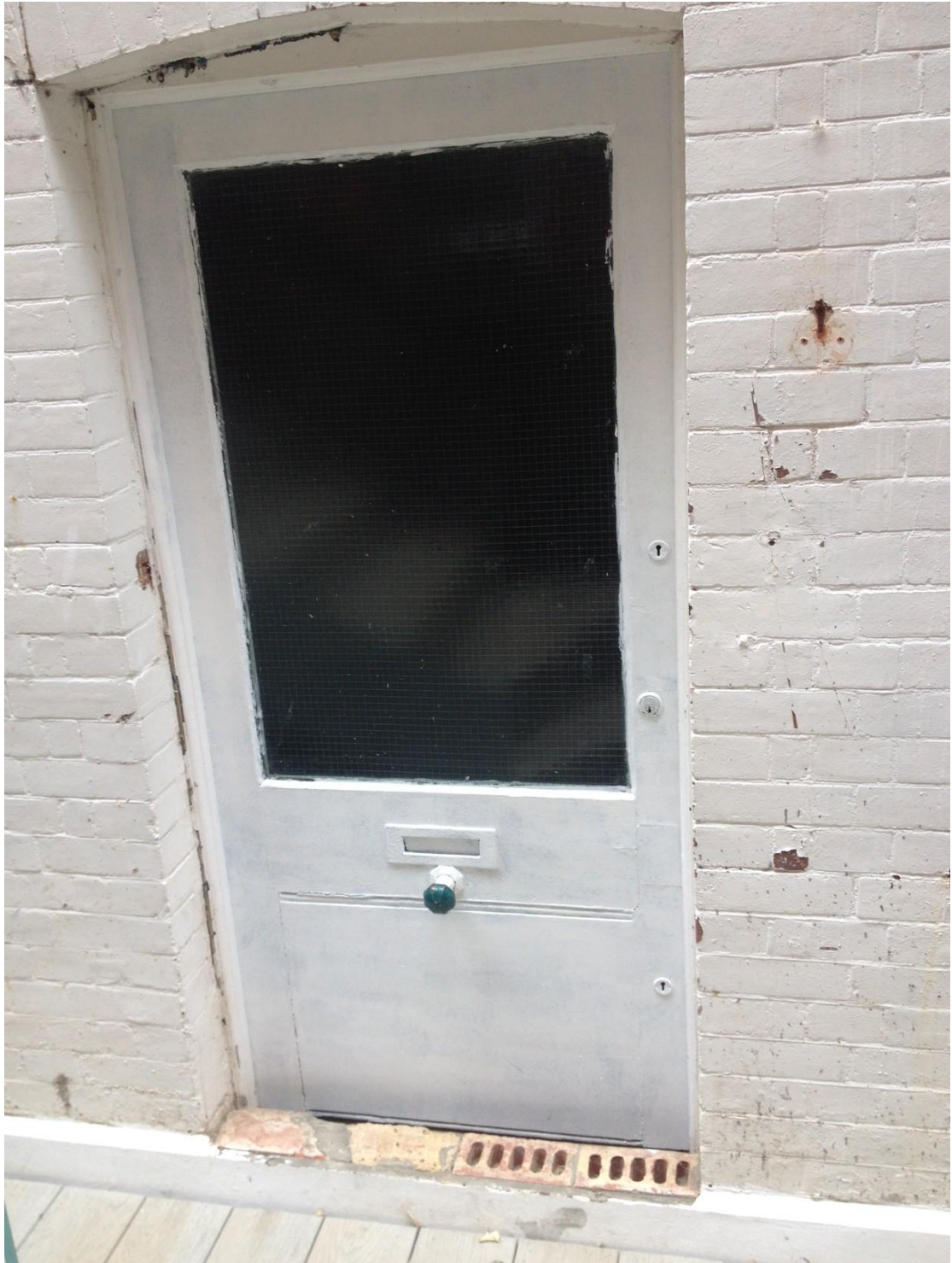
EXISTING SIDE (WEST) ELEVATION DOOR
