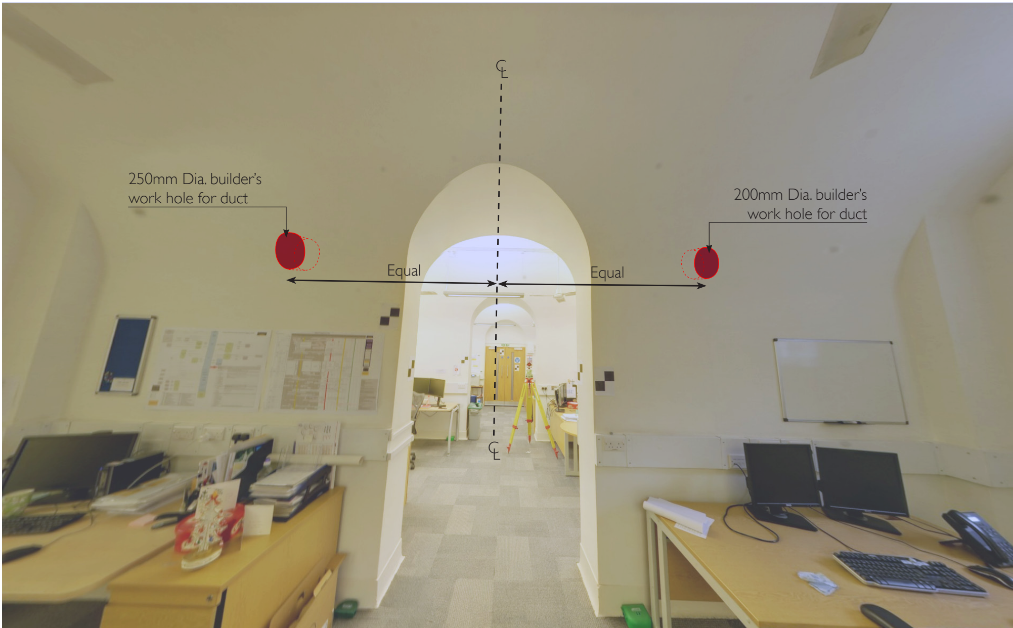
Indicative location of proposed builders work penetrations
