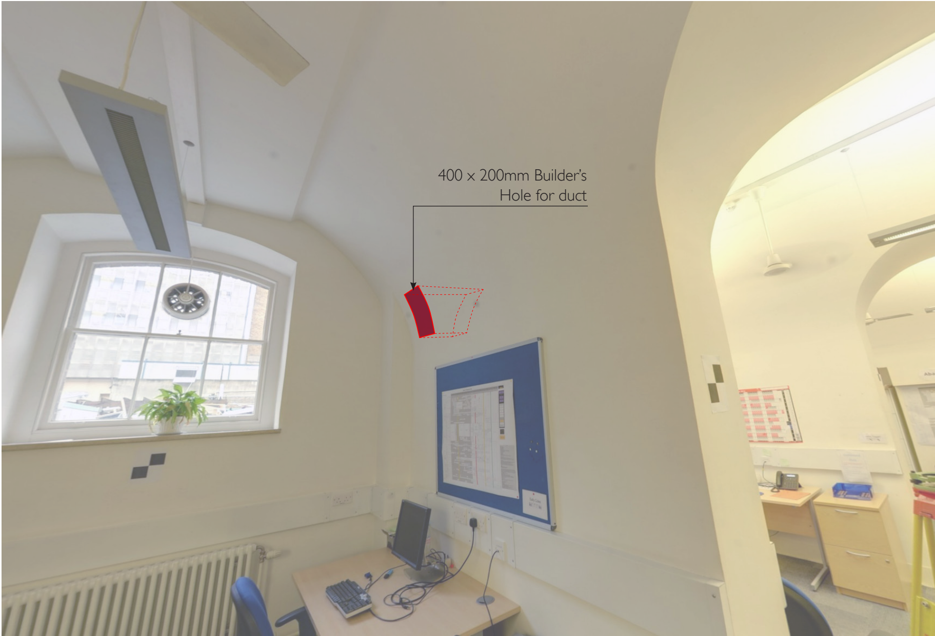
Indicative location of proposed builders work penetrations
