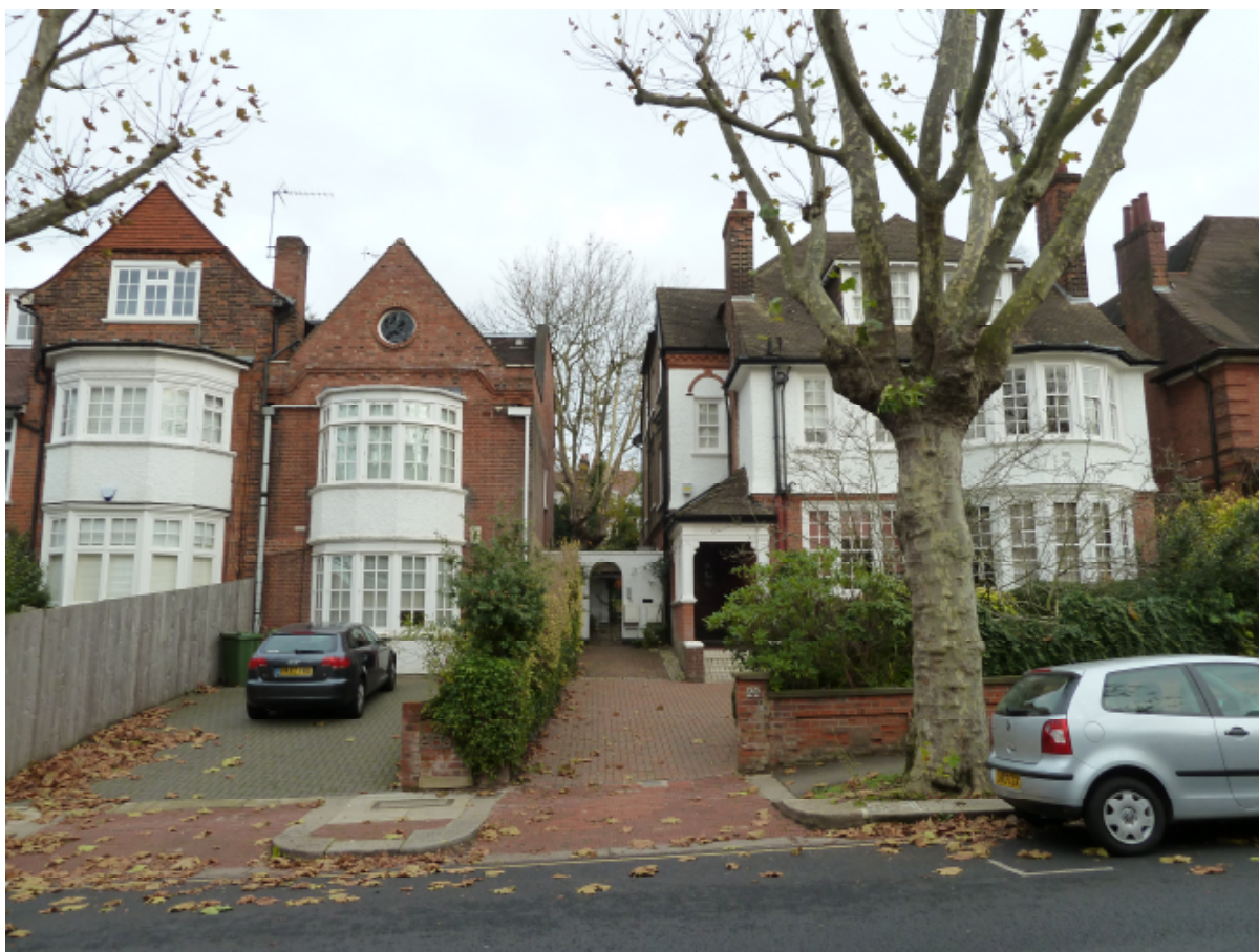
View toward front of property (showing location of proposed garage)
