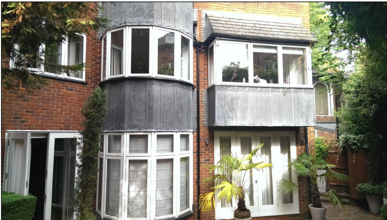
Figure 2: Rear of B1.
