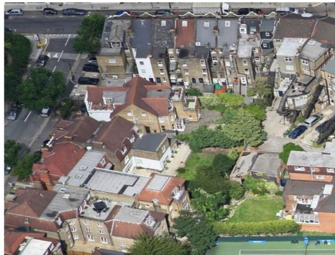
06 ARIEL VIEW OF REAR ELEVATION LOOKING TOWARDS THE EXISTING FLAT ROOF AND MANSARD ROOF
