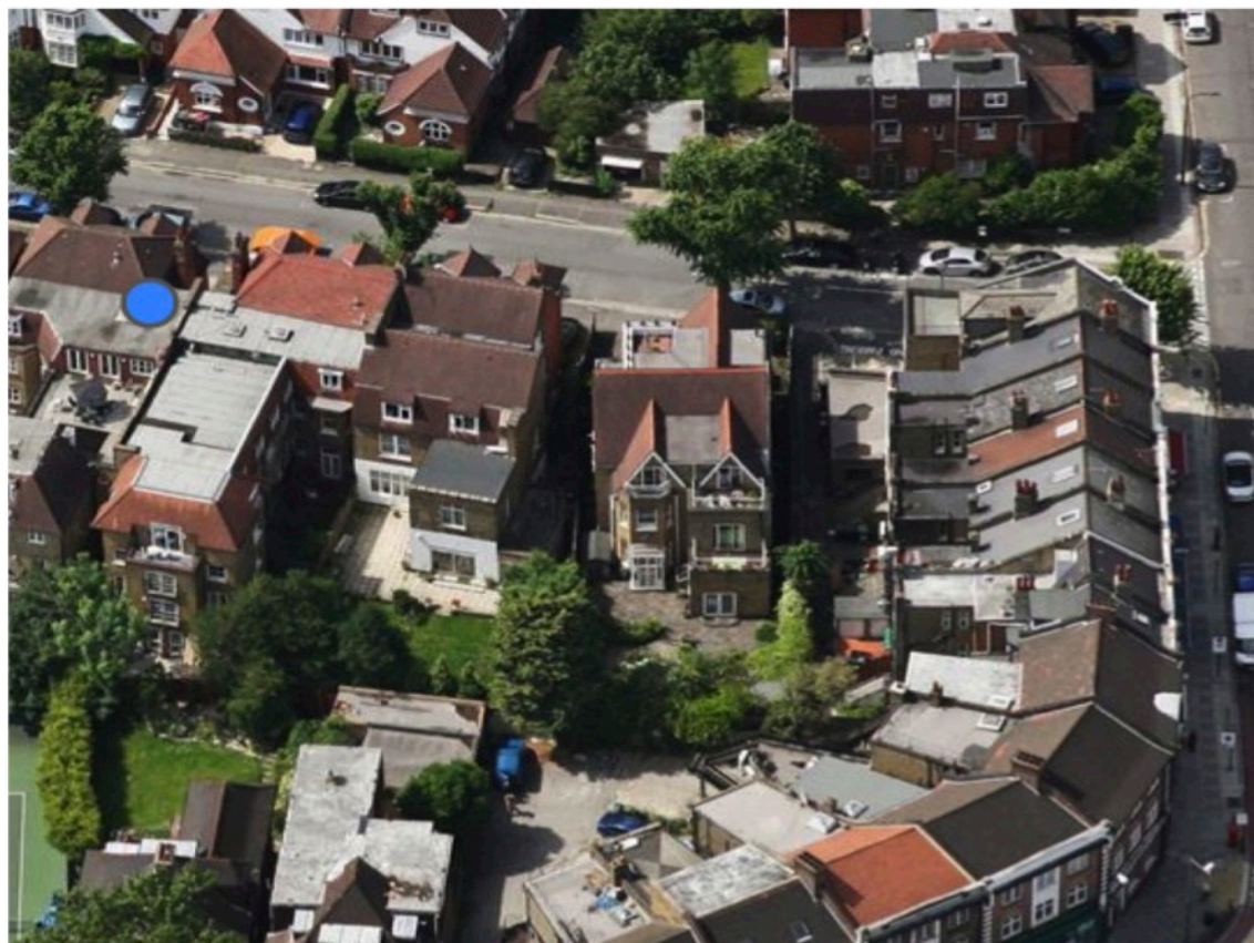
05 ARIEL VIEW OF REAR ELEVATION LOOKING TOWRDS THE EXISTING FLAT ROOF
