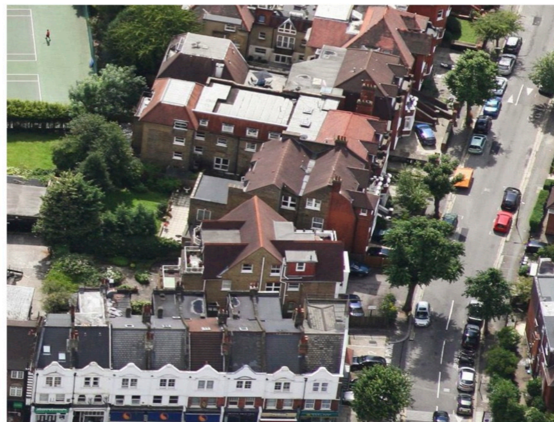
08 ARIEL VIEW LOOKING TOWARDS THE SIDE ELEVATION WHERE THE VALLEYS BETWEEN THE TWO GABLES CAN BE VISIBLY SEEN
