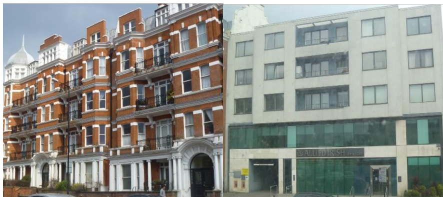
Images 005 and 006 – Examples of two buildings opposite the site which have balconies fronting onto Finchley Road
