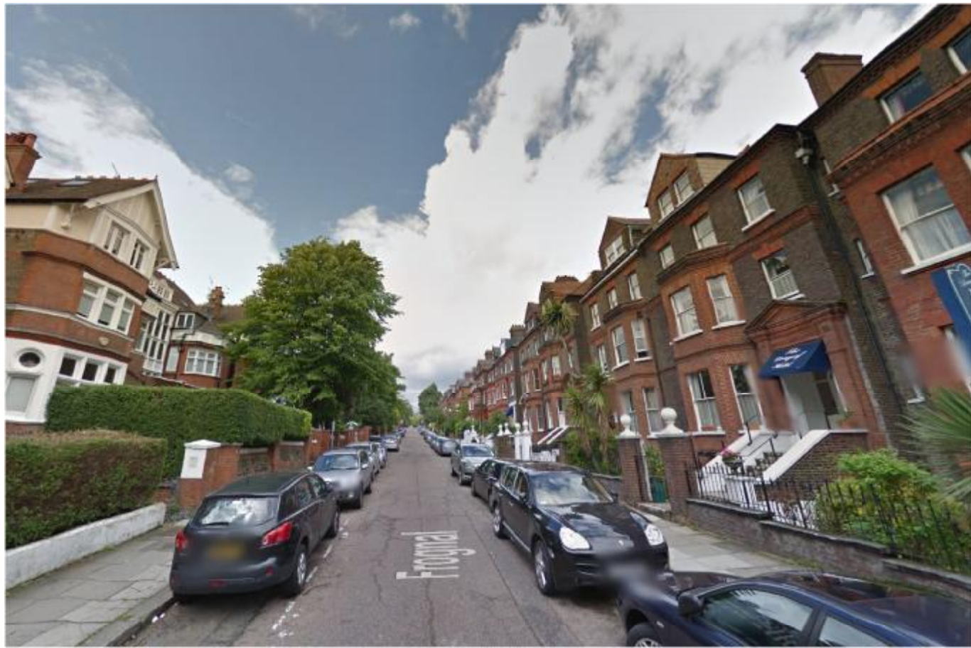
View facing North
