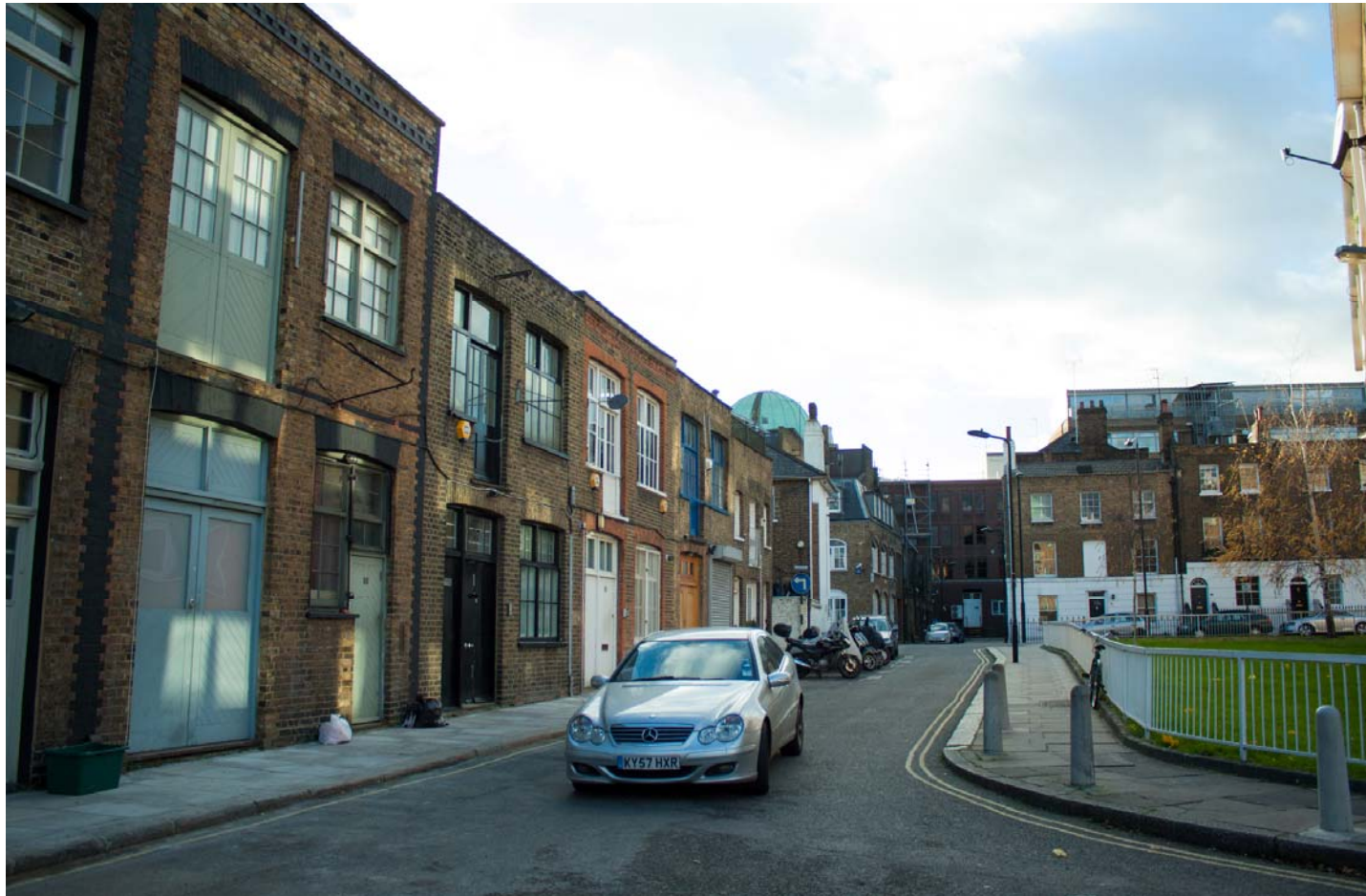
View towards Bayham Street facing West
