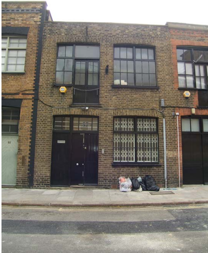
View of North elevation
