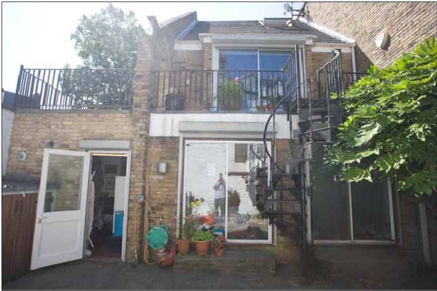
Rear elevation of main building
