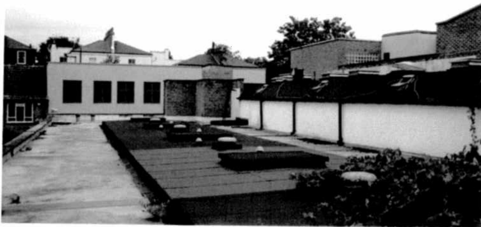
Photograph 3 – Showing the rendered façade and felt roofing.
