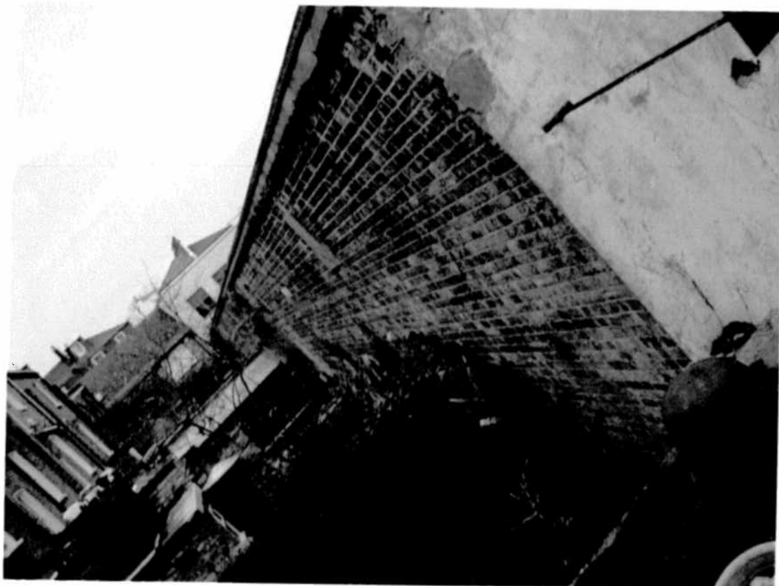
Photograph 1 – Showing the 4.5m high brick wall which will be retained.
