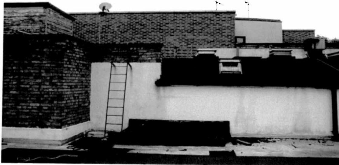
Photograph 4 – Showing the small area of brickwork and neighbours facades
