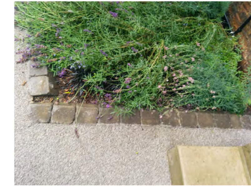
6 Existing brick planters 202_440 No Scale
