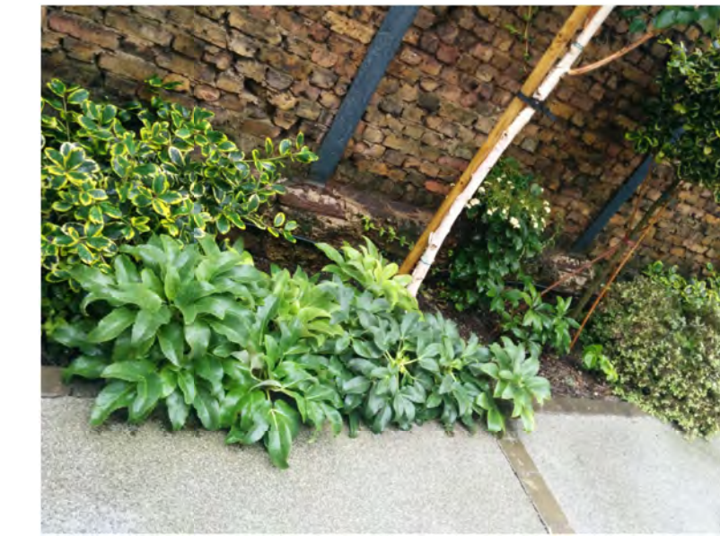
5 Existing brick planters 202_440 No Scale
