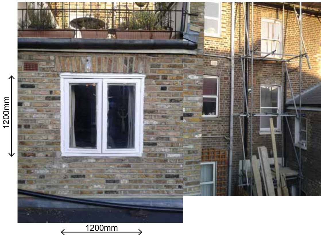
1. Existing back facade window.
