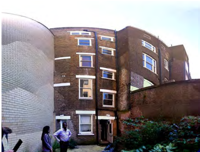
Fig 1.2.7 Rear condition of the property
