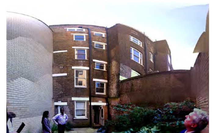
Fig 1.2.4 Rear of Guilford Street - Looking South
