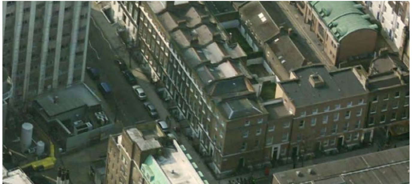
77-82 Guilford Street - Aerial view of roof
