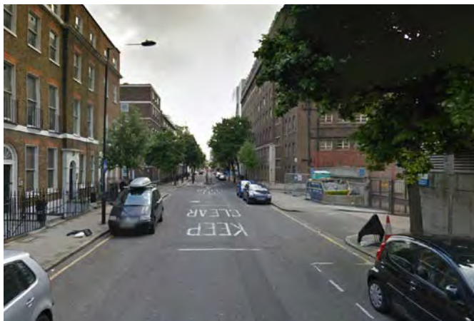
Fig 1.2.1 Guilford Street - Looking East
