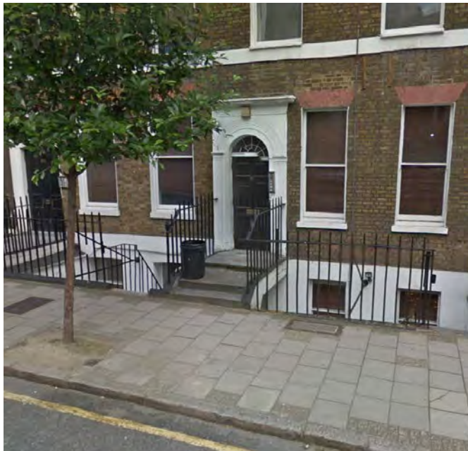
77-82 Guilford Street front access - Ground and basement levels
