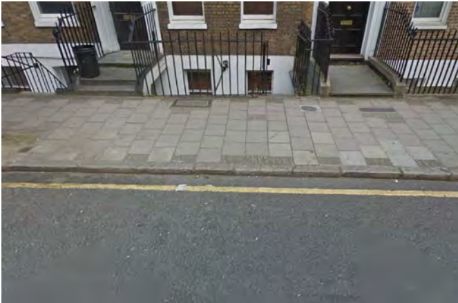
Fig 1.2.17 Pavement along Guilford Street
