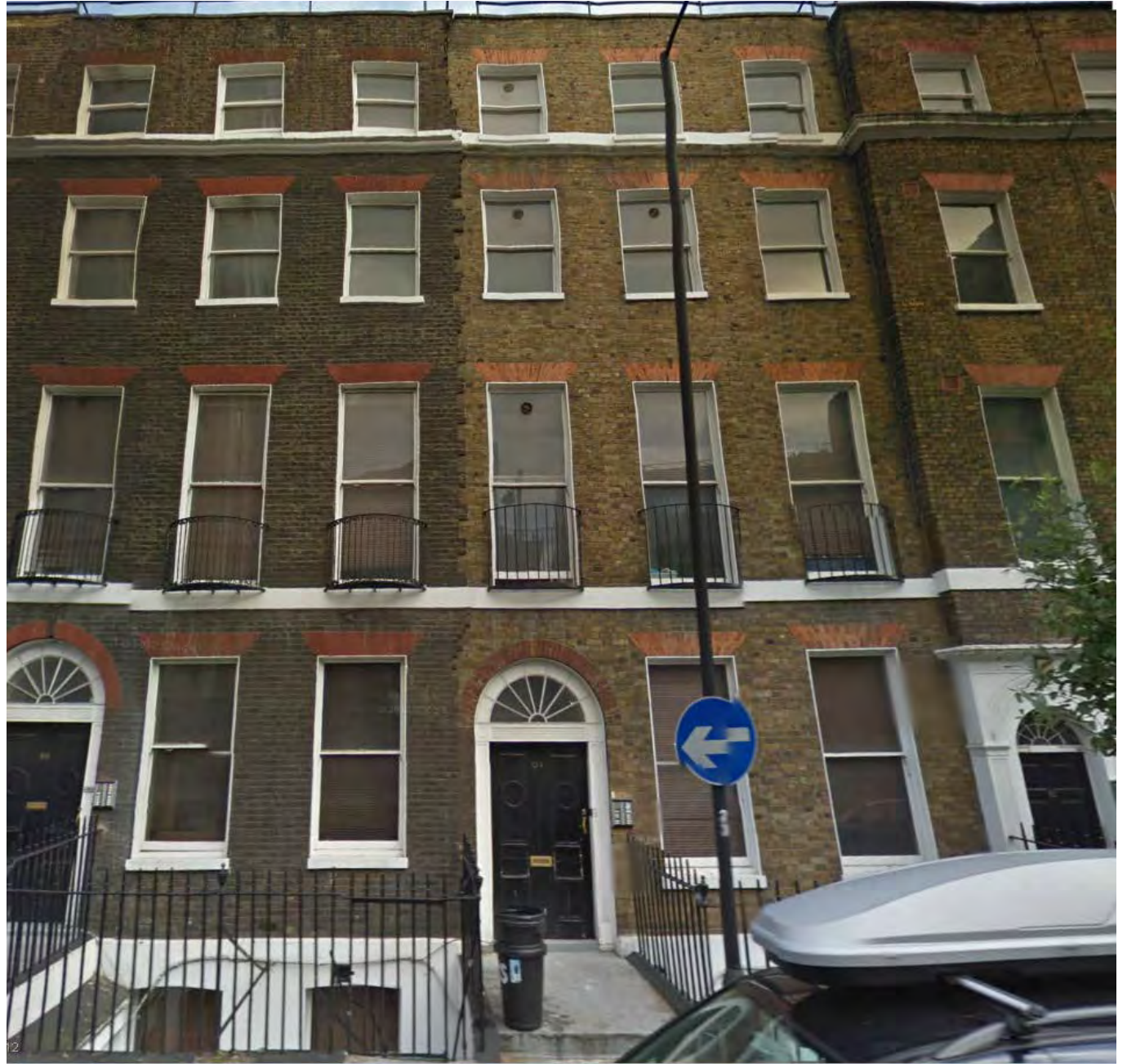
80-81 Guilford Street- Looking North
