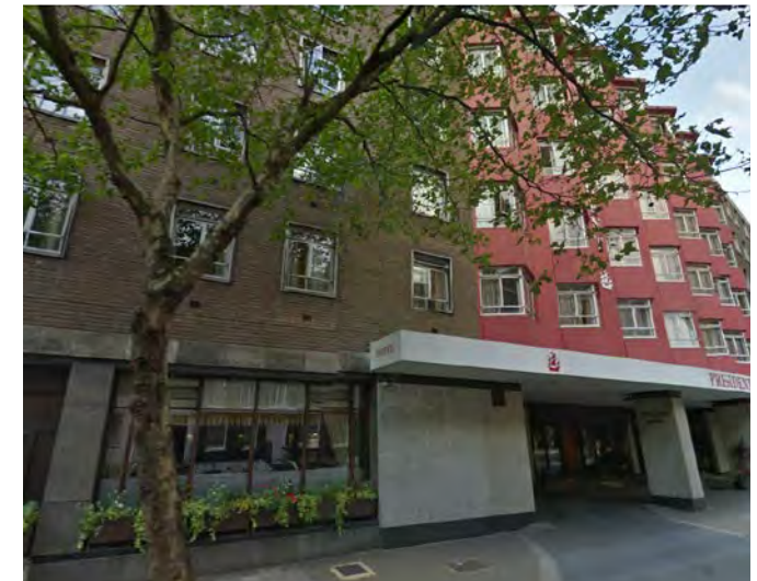
President Hotel from Guilford Street - Looking South
