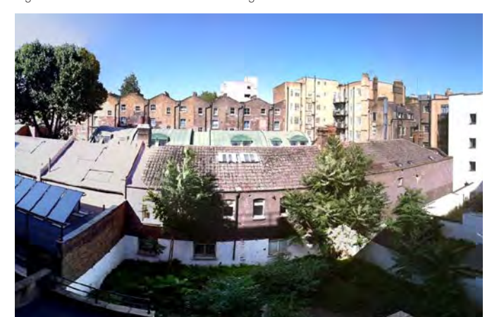
Fig 1.2.5 Rear of Guilford Street - Looking North
