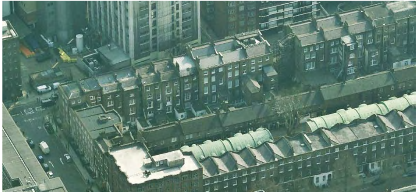
77-82 Guilford Street - Aerial view of roof
