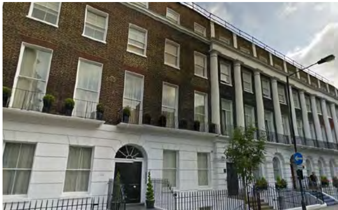
69-71 Guilford Street- Looking North
