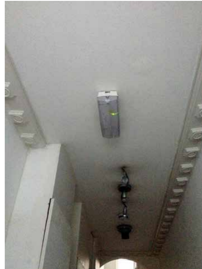
cornice to be retained / rebuilt as services boxing is removed
