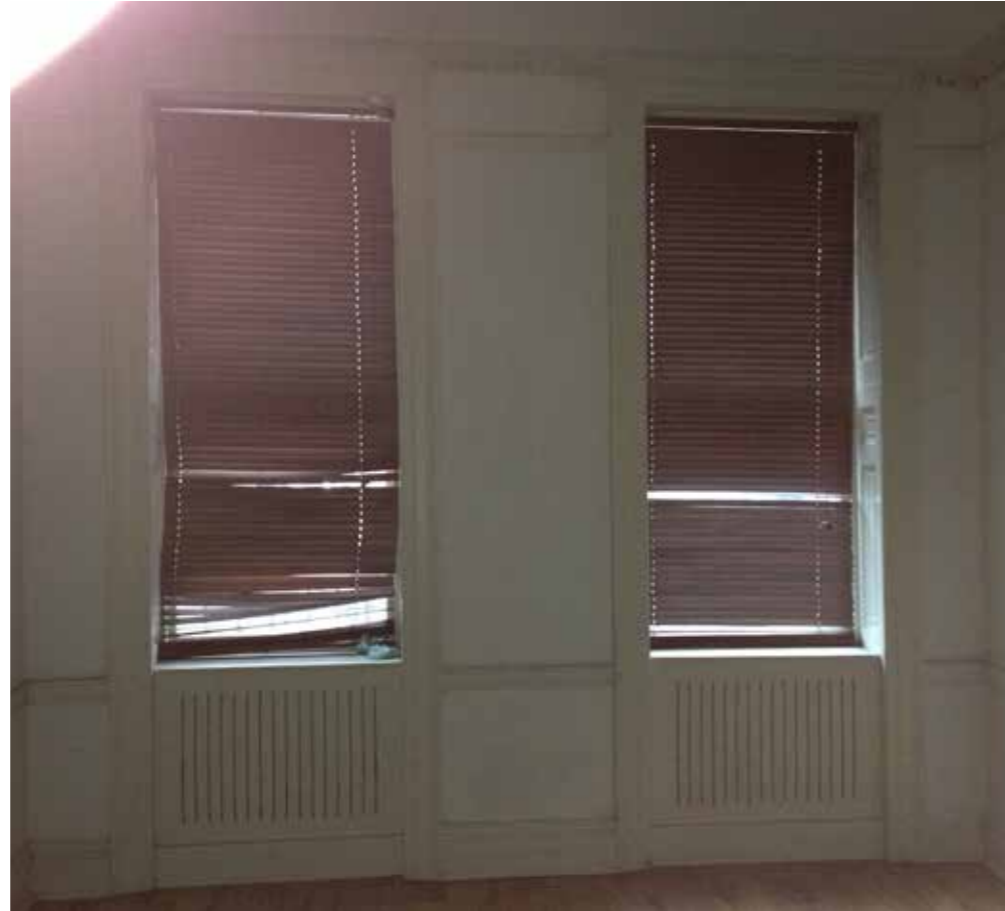
front windows to be restored as original
