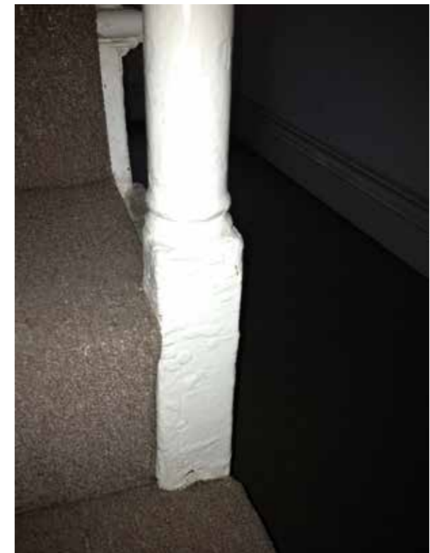
banister post detail to be retained
