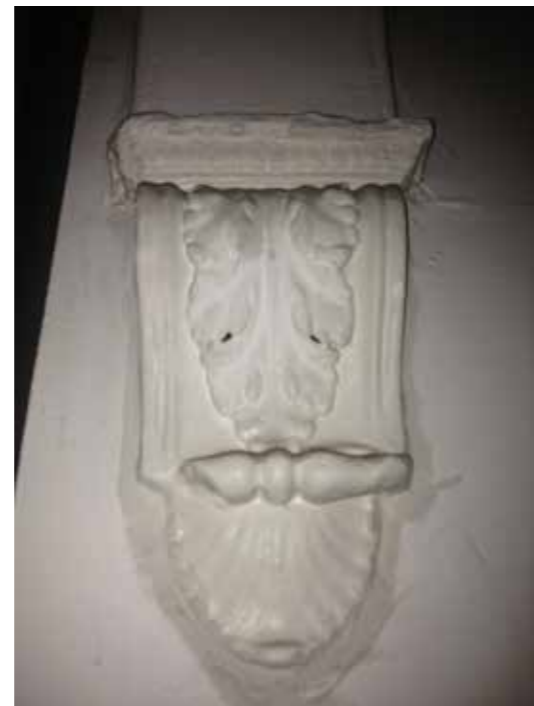
hallway arch moulding to be retained
