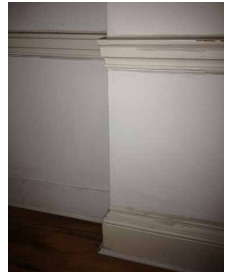
living room skirting and dado rail to be retained
