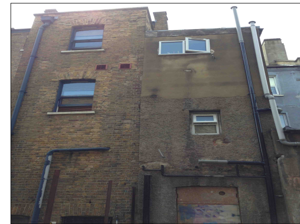
Photo Rear elevation- Existing
