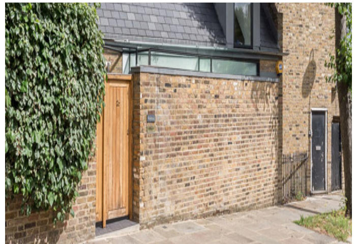
Detail of frameless entry glazing
