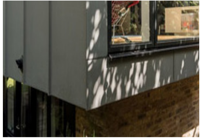
Detail of framed windows and zinc panelling
