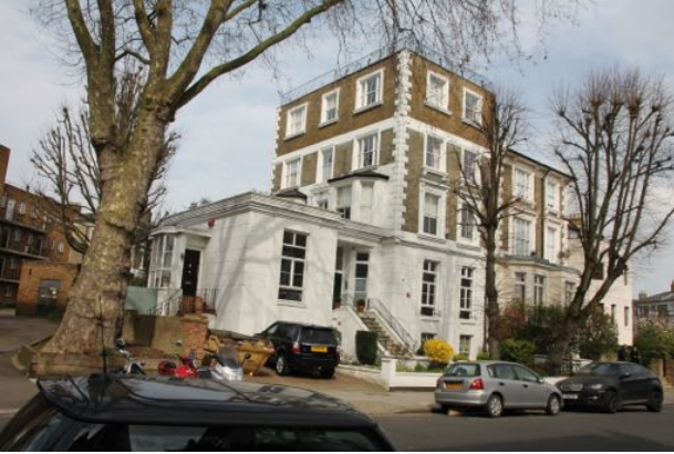
Front/flank view of 3 Upper Park Road. Flats 4 & 5 occupying top 2 floors & roof terrace
