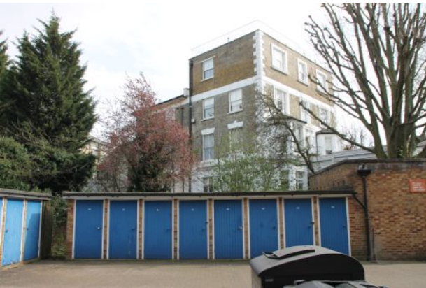
Rear/flank view from North West- Troyes House
