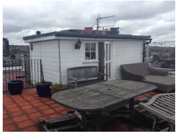
Stair building to roof terrace from South
