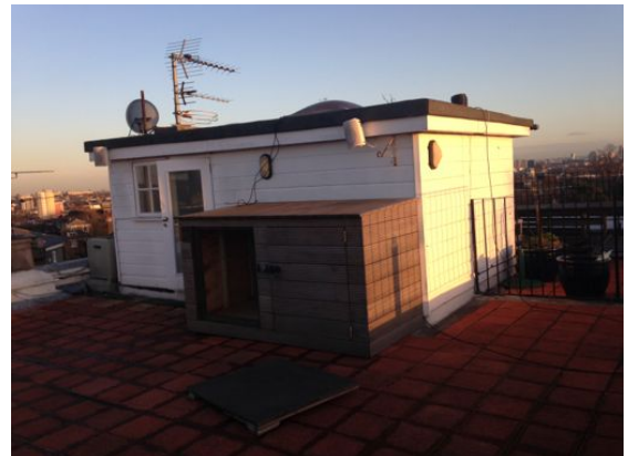
Stair building to roof terrace from North
