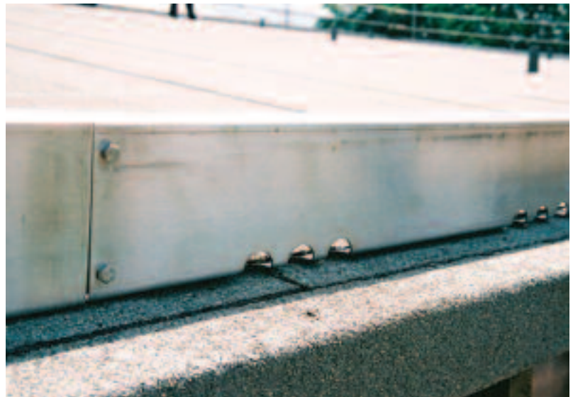
Icopal Stainless Steel Pitched Roof Edge Restraint
