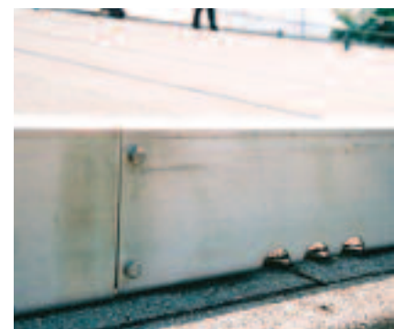
Icopal Stainless Steel Pitched Roof Edge Restraint
