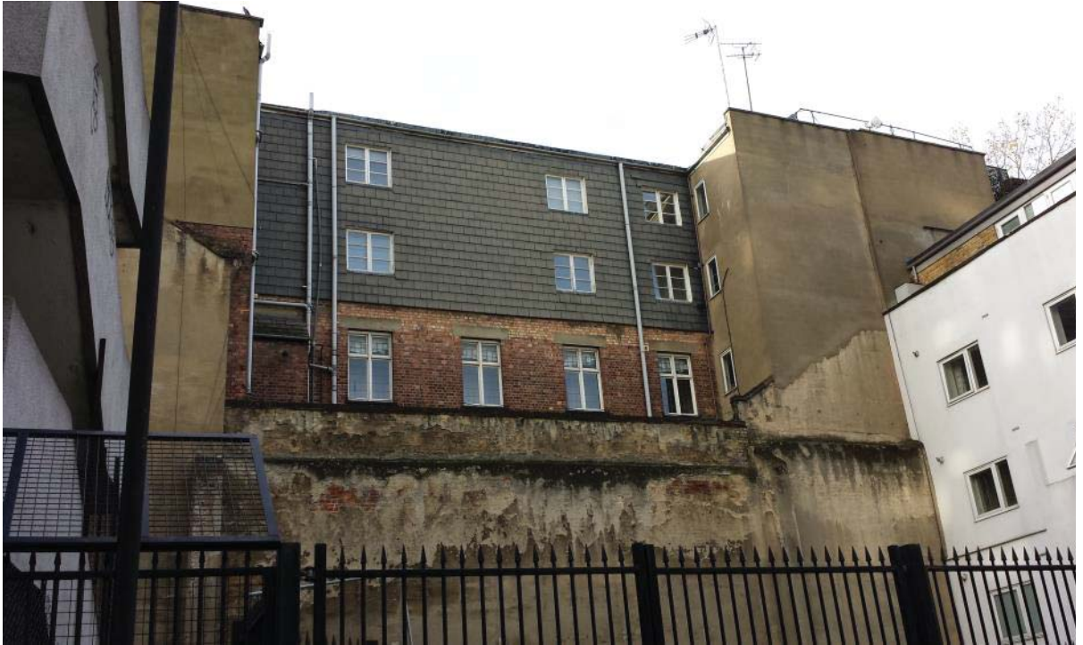
Figure 1437/F2 - Photograph showing the rear of 5-7 Grape Street
