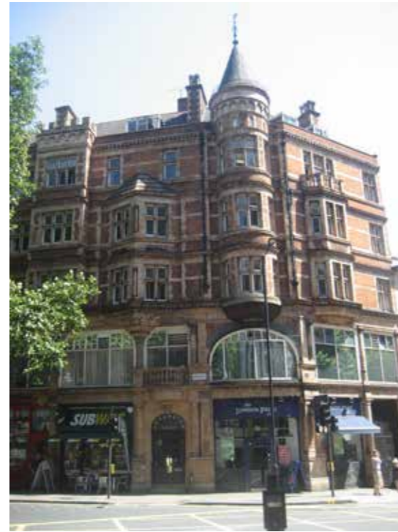
Fig. 6.7: Corner detail of Sovereign House on Shaftesbury Avenue.
