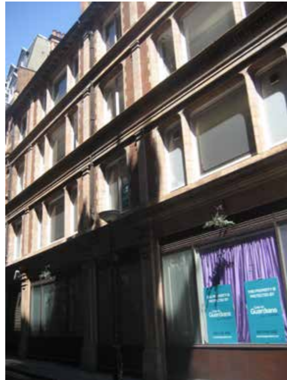
Fig. 4.20 & 4.21: 9-13 Grape Street facade.
