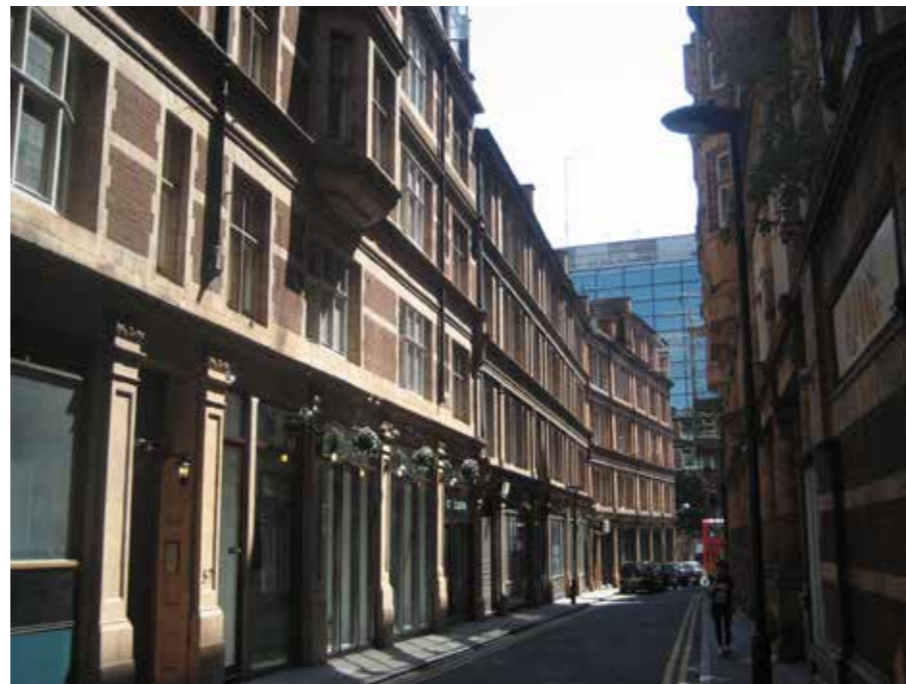
Fig. 4.24: Grape Street looking south. 9-13 is seen towards the centre of the image.
