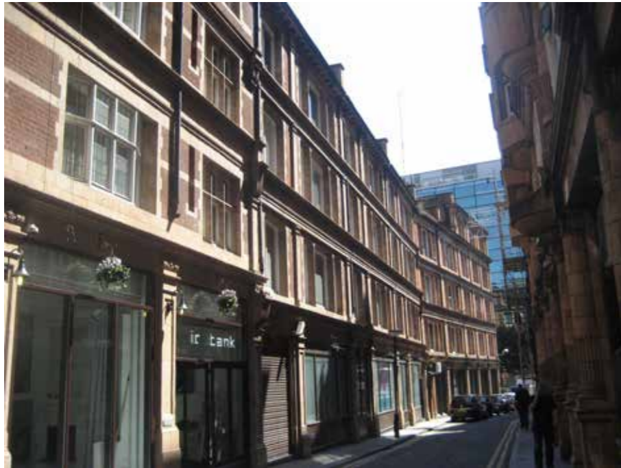
Fig. 8.2: (No. 1) 9 - 13 Grape Street, the subject site.
