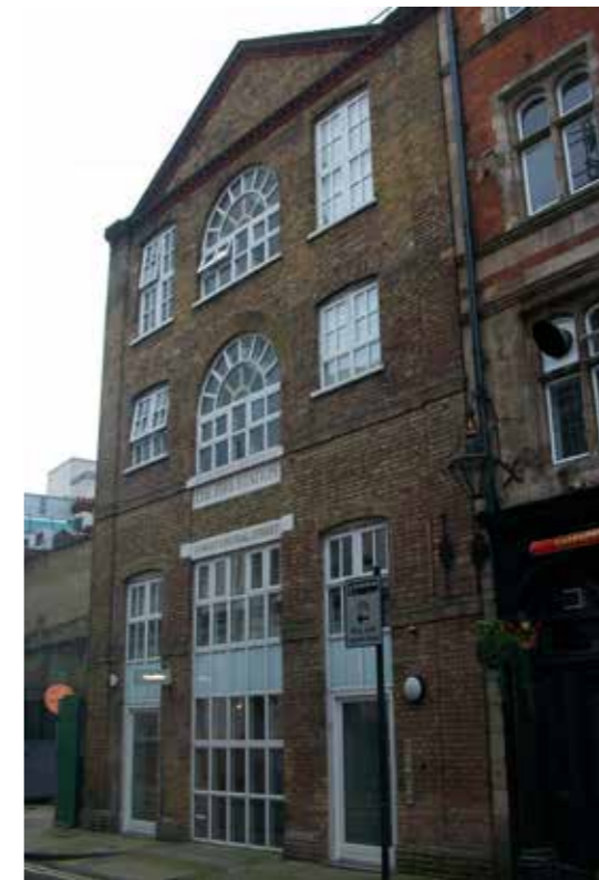
Fig. 8.7: (No. 6) 14 West Central Street neighbours the undeveloped space, seen to the left, beyond which is the rear of No. 9-13 Grape Street.
