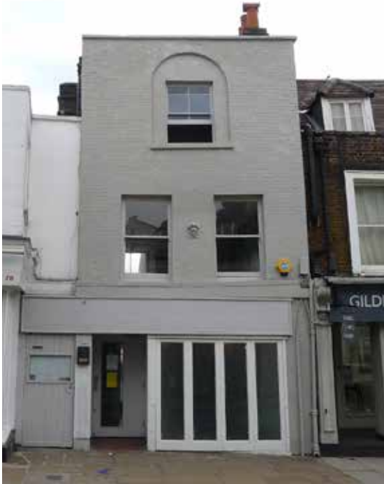
Part A - the principal, street front building showing 19thC facade, 21stC shopfront and alley way at left
