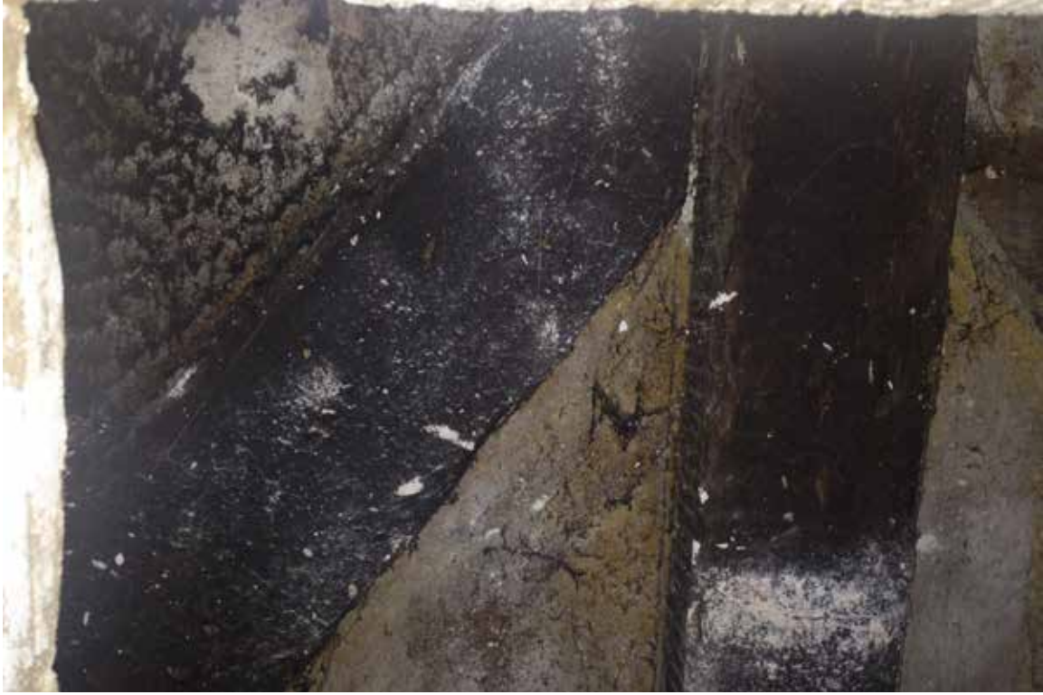
Fig 1: Investigation to the interior linings on the south boundary reveals old structural timbers with saw marks and hand-cut nails
