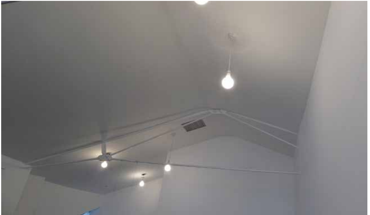
Fig xx: One of two existing steel trusses
